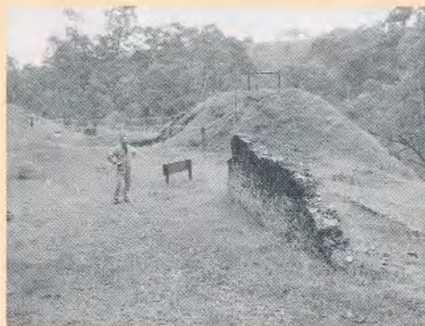
Main Shaft and winding plant ruins
